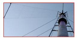
**TRAPEZOID ARRAY** - For use on industrial and commercial structures with guy ropes. Effective even if not the highest point.
