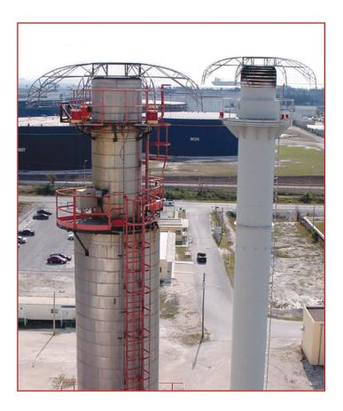
DAS interrupts the formation of these upward streamers through *point discharge,* a phenomenon where a well- grounded point exchanges ions between the air and the ground.
