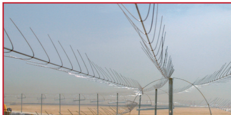
Rim Array Designed for floating roof tanks used in petrochemical and flammable storage industry.
