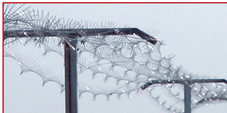
Paragon Array Multiple use configuration. Variant commonly used on transmission and distribution lines.
